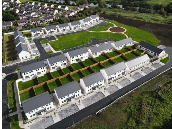
Rehins Fort, Ballina Completed September 2023
